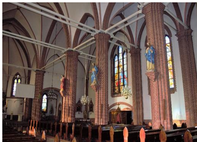
Fig. 6. Bytom-Karb. Church of Good Shepherd. Interior view from the center of the nave towards the north aisle. Visible inter-nave pillars with figures of the apostles, decorative brick cladding, pointed window openings, vaults, and steel reinforcements under the vaults.
