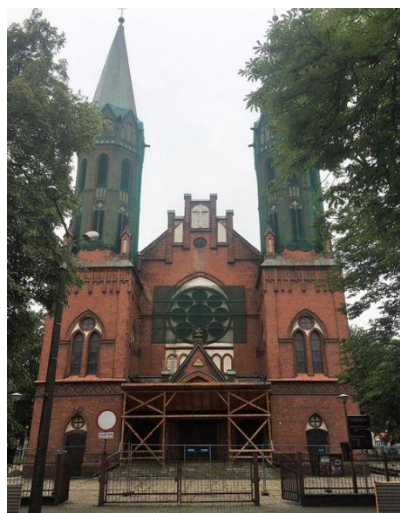
Fig. 2. Bytom-Karb. Church of Good Shepherd. View of the facade. The photo was taken during the protection of the upper parts of the towers and the main entrance to the church against further degradation due to mining damage. Source: own photo
